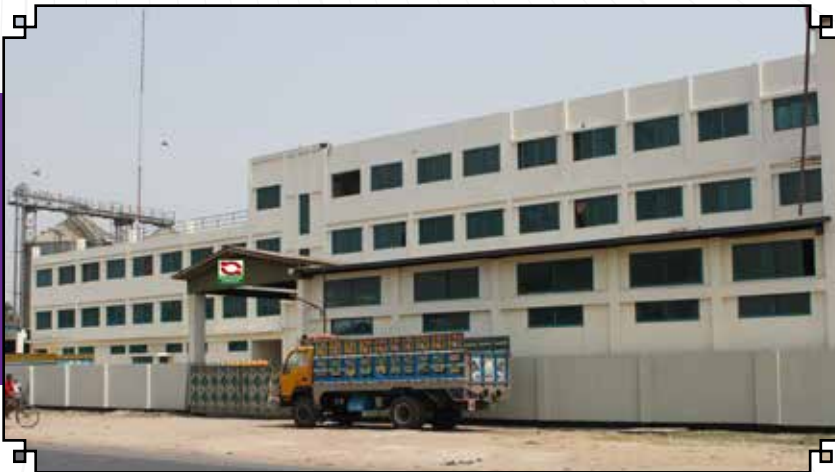
Photograph of the National Feed mill Ltd, Financed by Meghna Bank Ltd.
